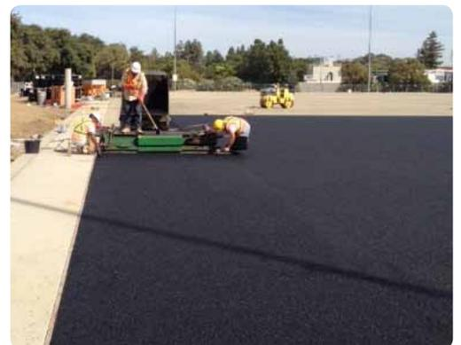
The team of Rec-Turf and Polytan installation technicians are shown here installing the in situ (paved directly onto the sub-base) Poly-Shock Pad underlayment at Dairy Outdoor Recreation Complex.
